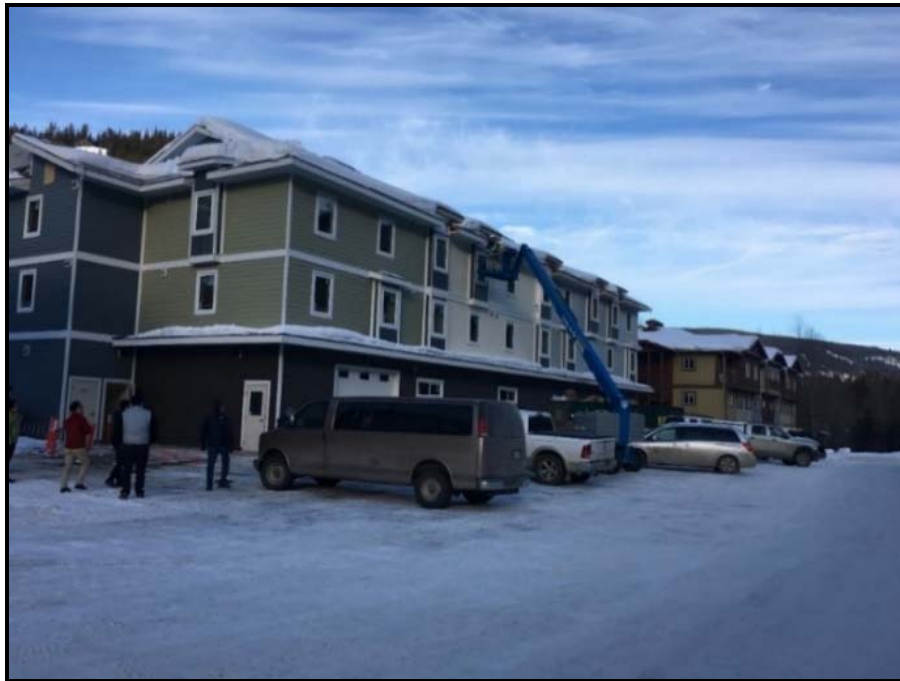
Construction of the Big Bear Lodge Employee Housing
