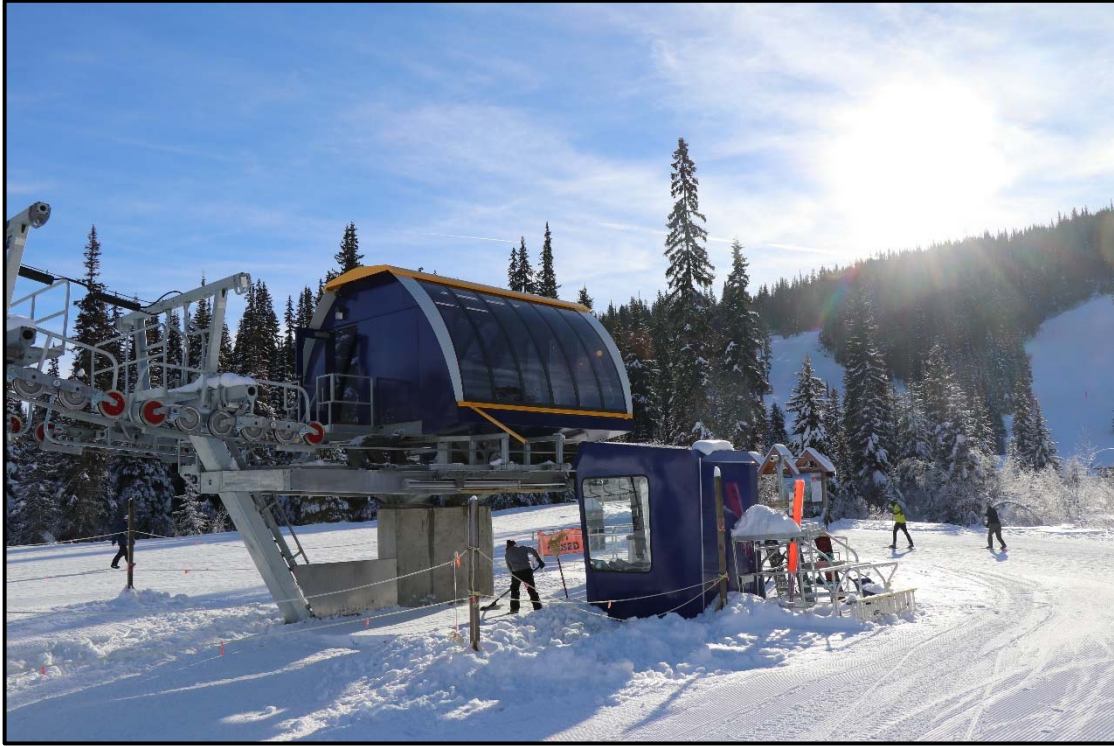
Orient Quad Lower Lift Terminal
